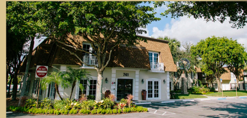
GLOBE OFFICE PROJECT
